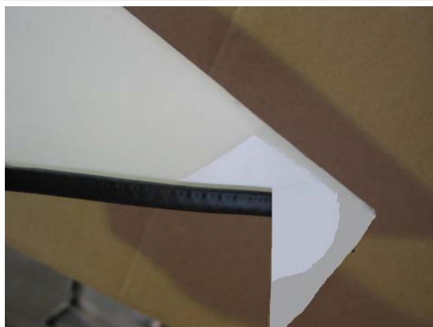
Figure 7: 3mm clip lock, trimmed to suit rear of cut off
